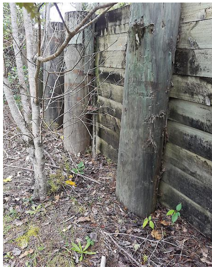
Figure 28. Timber pile wall.
