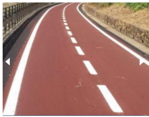
Figure 10: Red Coated Asphalt (P.E. Phelan et al., 2017)
