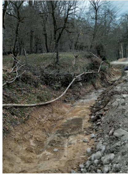
Figure 13. Removing Sludge and sediments, reviving the existing roadside ditch
