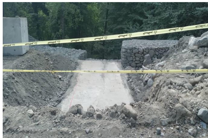
Figure 10. An example of preparing the placement of prefabricated concrete Culverts
