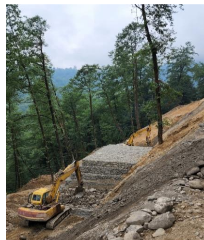
Figure 26. Gabion retaining wall km:3+200.
