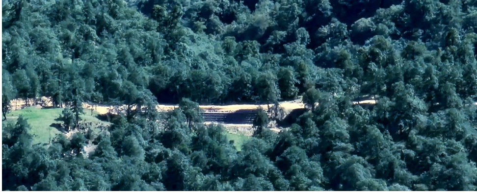
Figure 32. Retaining wall seen from the mountain peak, Km: 6+050
