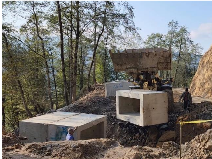
Figure 11. Placement of Culvert boxes
