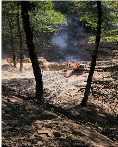
Figure 29. Retaining wall construction km 7+500
